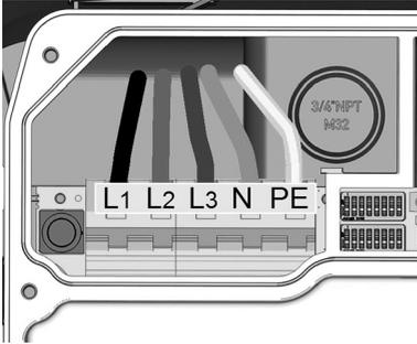
1. Cut the connecting wires to the appropriate length. They should be kept as short as possible.
